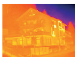
Image thermique sans testo ScaleAssist
